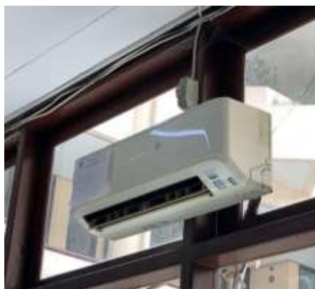
Gambar 3. AC split konvensional ½ PK 420 watt
